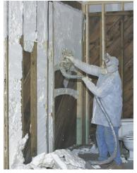
An improperly insulated attic or damp basement can lead to problems with indoor air pollution, including mold and mildew, says Atlanta remodeler Jerome Quinn. Green products and techniques such as spray foam insulation, radiant roofing panels, caulking foundation joints and sealing off crawlspaces help to eliminate these problems at their source. "Creating a healthy interior living environment and energy efficiency go hand in hand," he says.
