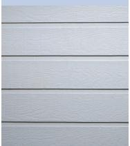
Bishop knows his stuff when it comes to siding. "We use (James Hardie) Hardiplank siding when we can on our projects. It is a durable no-rot product that virtually lasts forever. It is immune to water and termite damage. It blends with other siding materials so it can be put on an addition without interrupting the 'flow' of the house. It is non-combustible; contains no formaldehyde, fiberglass, or asbestos, and has a 50-year warranty." www.jameshardie.com
