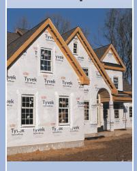
For exterior protection, Gardner/Fox relies on an industry mainstay. "Tyvek housewrap is a product that we have been using on homes for a number of years. Installed properly this product performs very well with stopping air flow through wall cavities and keeping out wind-driven rain, but still allows moisture vapor to escape from inside walls."
